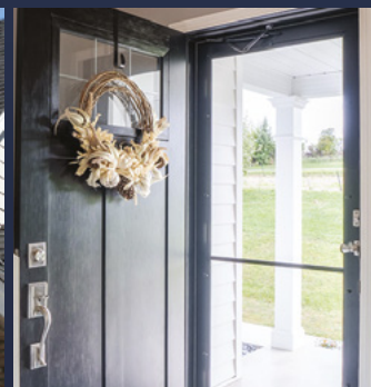
ENTRY DOOR REPLACEMENT
